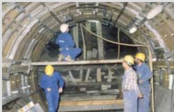
Figure 3.27 The three types of lining so far used in the underground facility. At the top: nodular cast iron segments (HADES experimental gallery); in the middle: concrete segments (small gallery and Test Drift); at the bottom: sliding steel ribs (Test Drift, ANDRA section).
