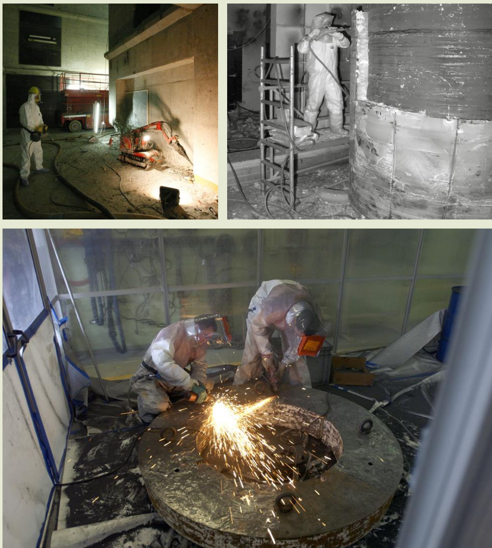
Figure 19 – Above: dismantling of the Eurochemic pilot reprocessing plant (source: Belgoprocess and Bonsei Publicatiebureau); below: dismantling of part of the BR3 research reactor (source: SCK•CEN).
