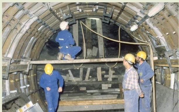
Fitting the lining at the end of the second gallery, called "Test Drift"
