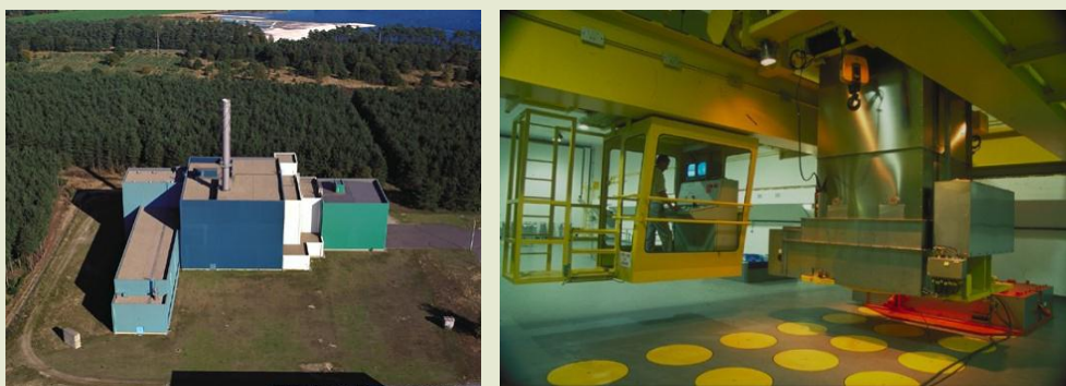
Figure 16 – External and internal views of building 136 of ONDRAF/NIRAS operated by Belgoprocess intended for the storage of high-level and medium-level conditioned waste. This building has been designed to withstand extreme external conditions such as earthquakes, explosions and military aircraft crashes. The containers of category C waste, which are handled remotely from a shielded control room, are stacked in silos equipped with a ventilation system designed to remove the heat that they emit. For each 450 kg container, this heat is initially comparable to that of a domestic electric radiator with a power of 2000W (source: Belgoprocess).
