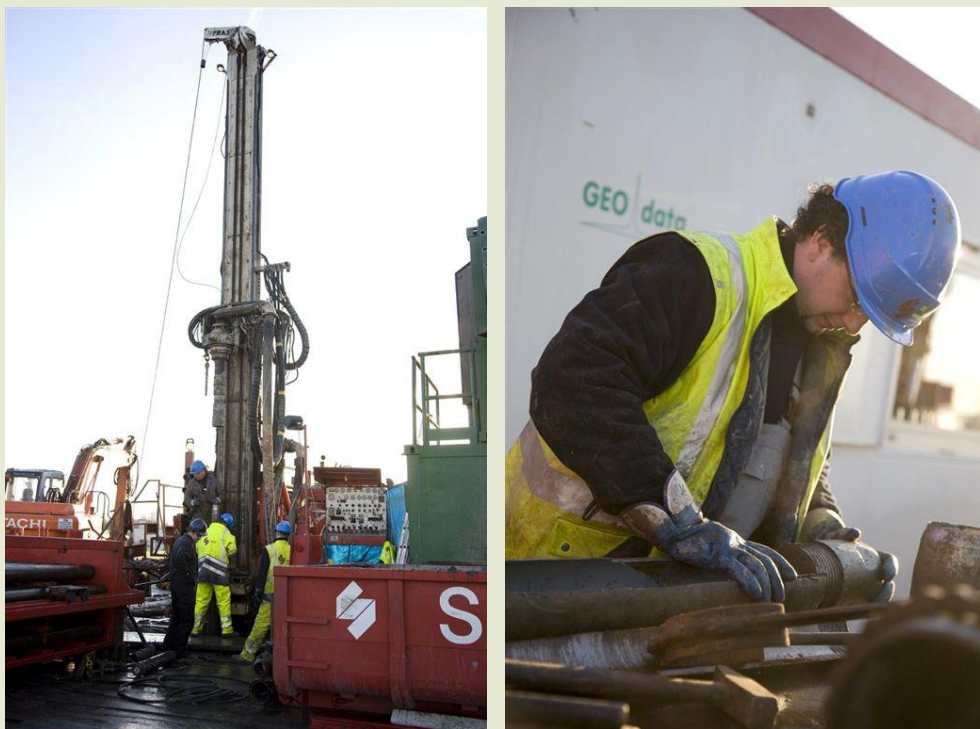
Figure 43 – Exploratory drilling and core drilling for Ypresian Clays at Kallo.
