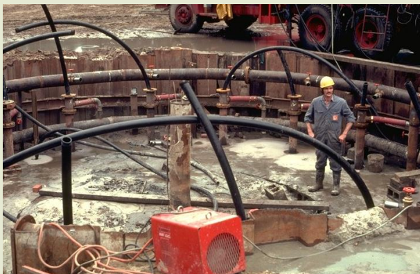
Freezing the soil with a view to constructing the first shaft
