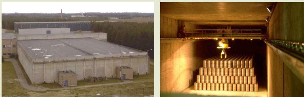
Figure 15 – External view of building 127 of ONDRAF/NIRAS operated by Belgoprocess designed for the storage of medium-level conditioned waste, and an internal view of one of its four bunkers. The waste is handled using a travelling crane controlled from a separate control room (source: Belgoprocess).
