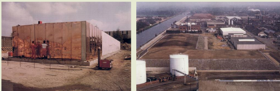
Figure 48 – Umicore’s UMTRAP licensed interim storage facility in Olen. Left: placing of the copper confinement barrier over a concrete bunker; right: overview of the site after the covers have been installed (source: Umicore).
