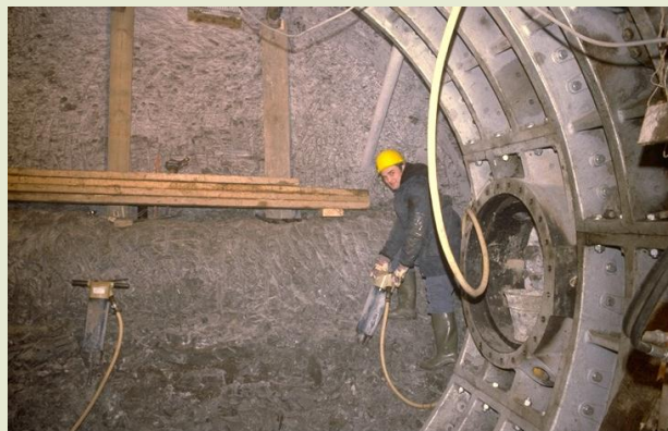
Excavating and fitting the lining of the first HADES gallery
